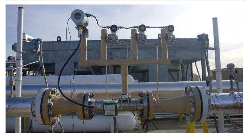
The higher liquid surface tension means the flow through the VorCone meter can't be modelled as homogenous, a data fit is required.
