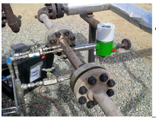
• 2" VorCone Meter installed at saturated steam oil well injection point. (82 Bar)
